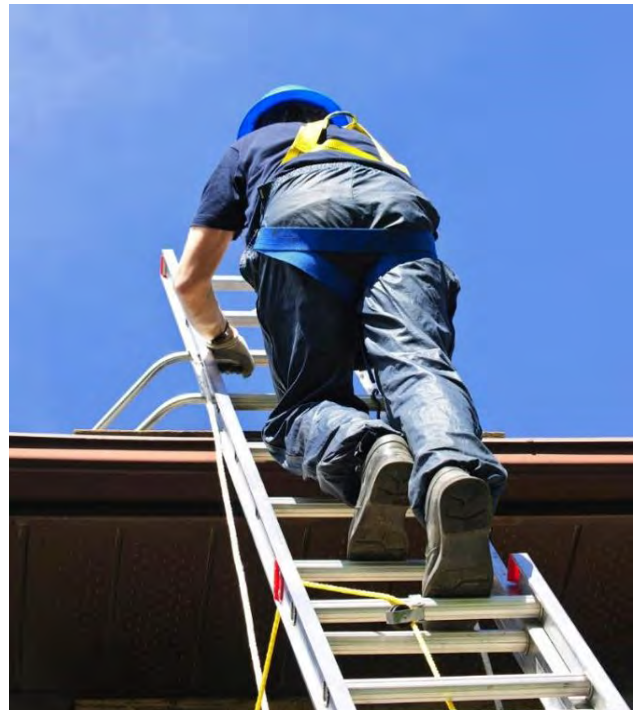
Maintain three points of contact when using ladders.
