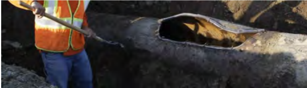
Over-pressurized equipment can lead to incidents, serious injuries, or death.
